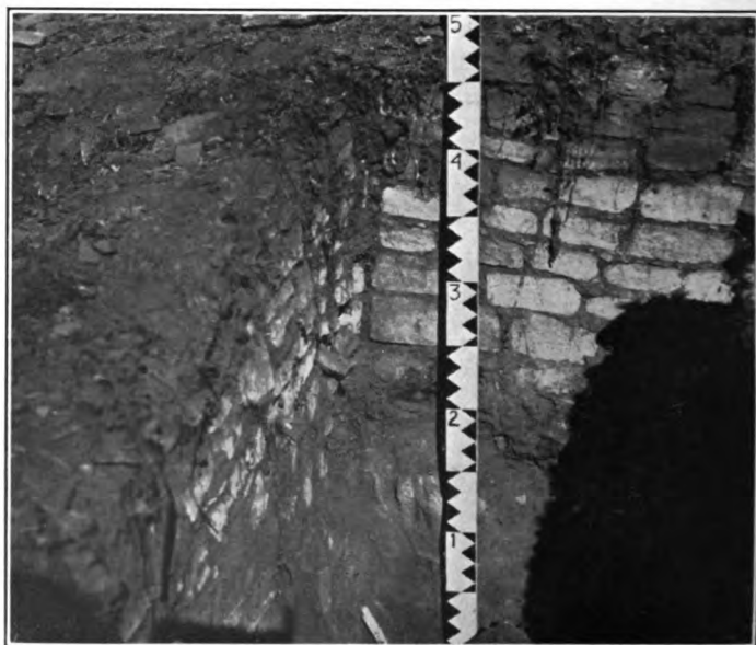
b. Difference in foundation levels between old and later sections of building
